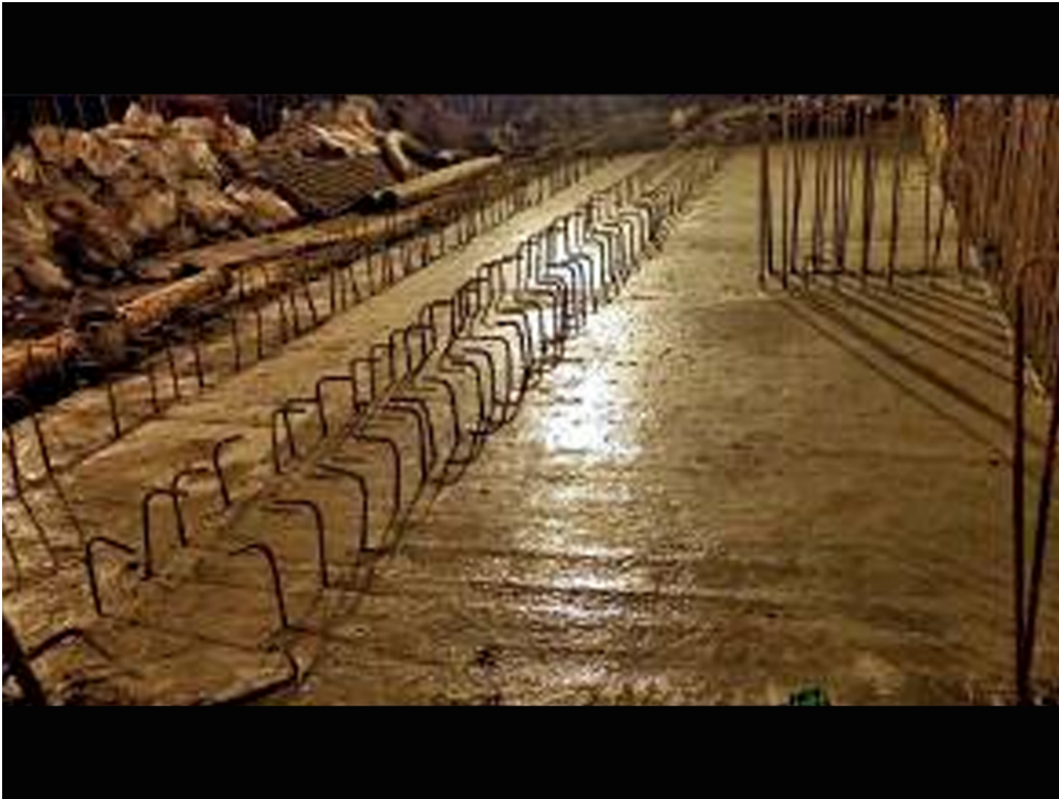
The base slab, which was completed over the weekend
